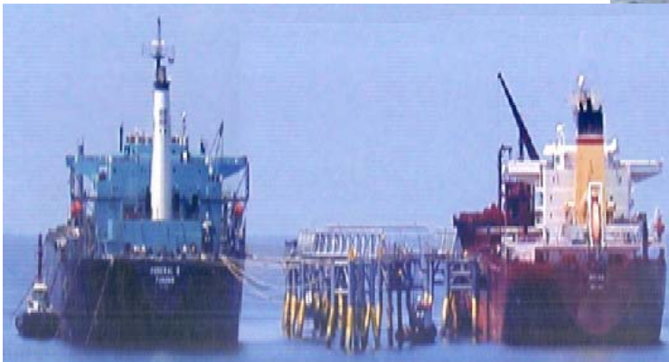
Condensate Offloading Terminal
