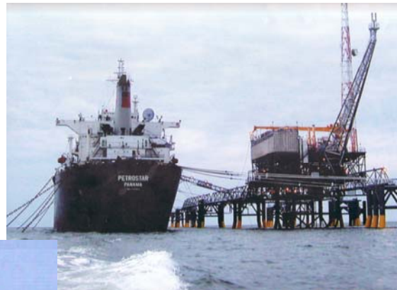
LPG Offloading Terminal
